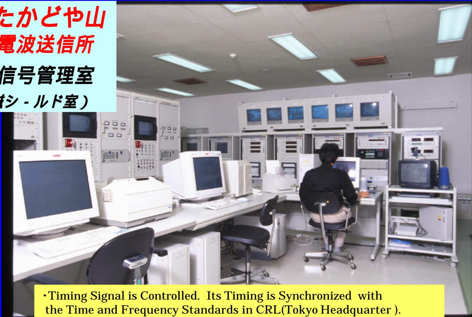
• Timing Signal is Controlled. Its Timing is Synchronized with the Time and Frequency Standards in CRL(Tokyo Headquarter).
